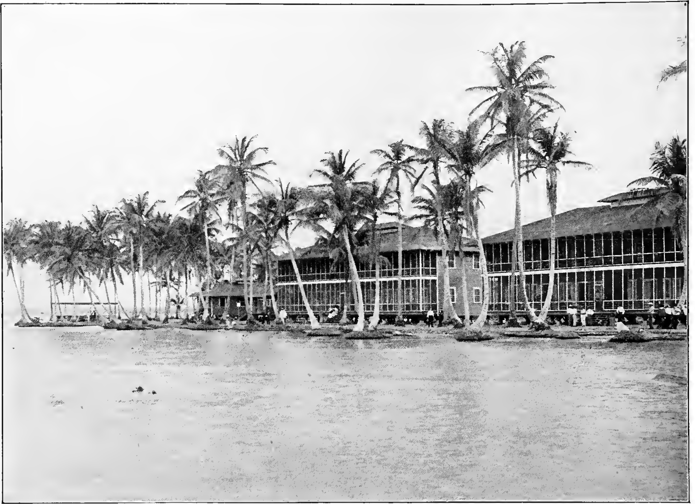
BACHELOR QUARTERS AT TORO POINT
